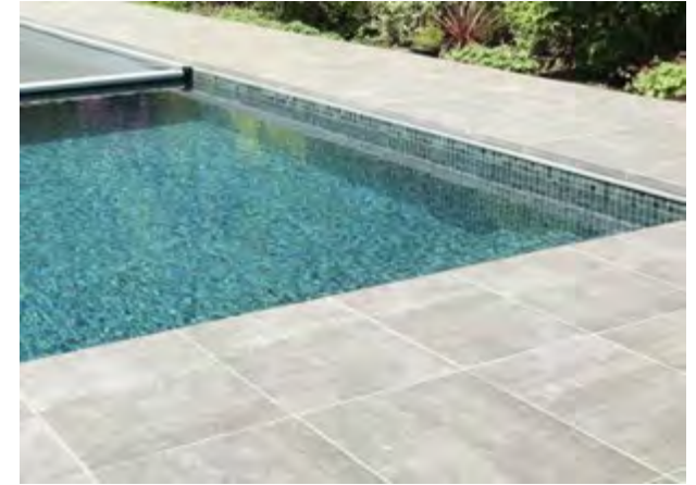
Porcelain Over-lip coping with automatic pool cover system
