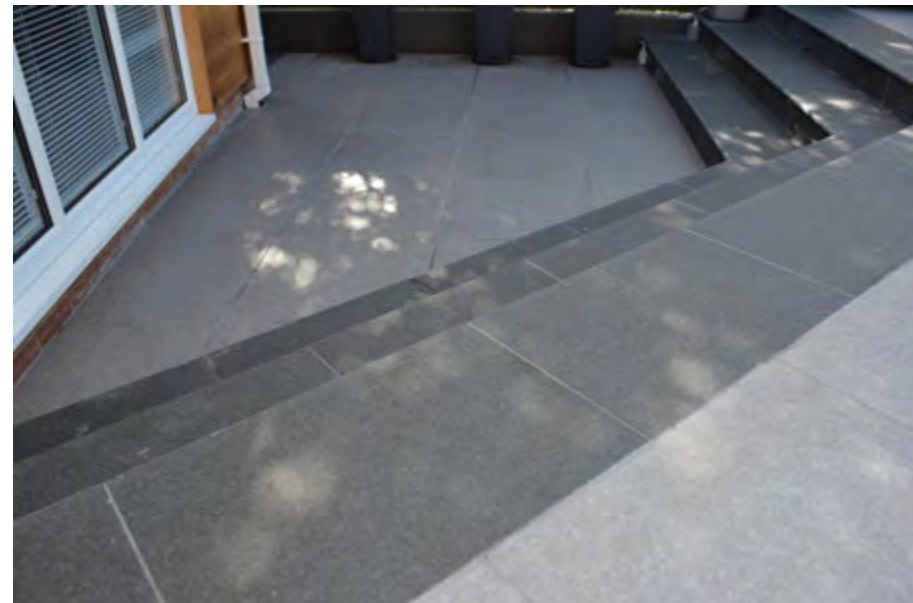
Boston Bespoke steps with Namur paving
